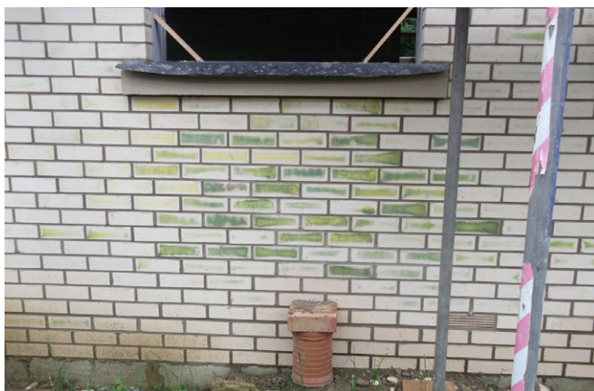
Vanadium staining visible on a light brick
