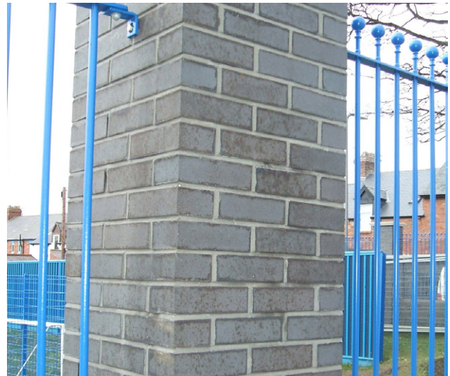
Peacocking is unique to blue brick
