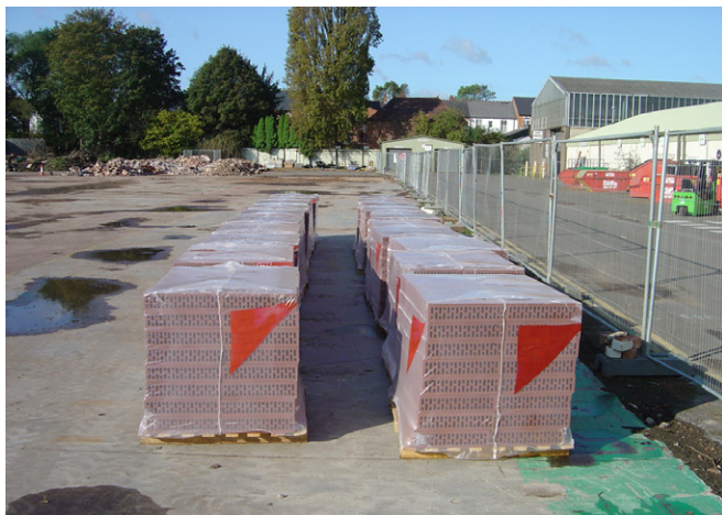
Stored bricks must be protected from inclement weather.
