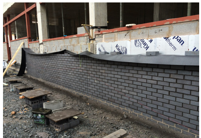
Bricks protected from rainfall, including stacks.
