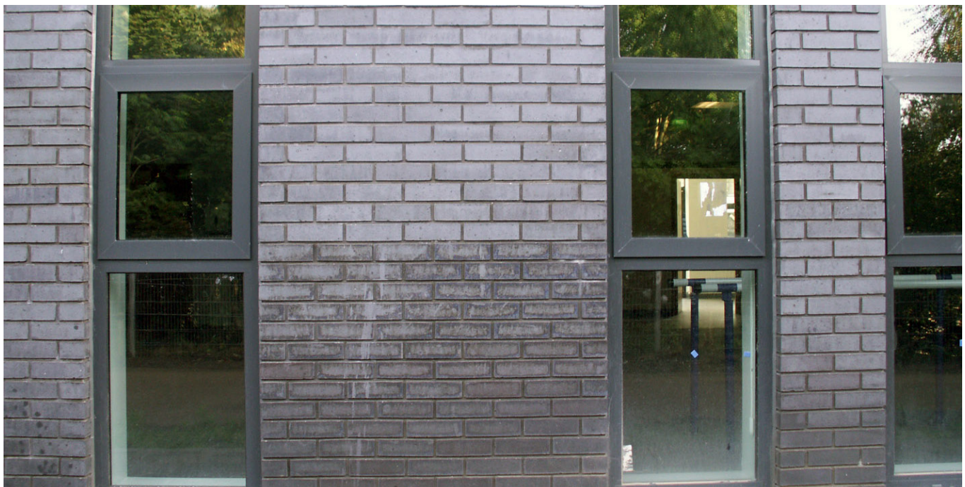
Picture framing likely due to saturation during construction
