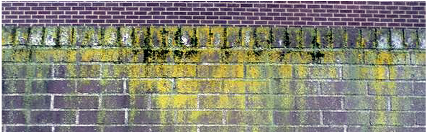
A coping detail could have reduced dampness.
