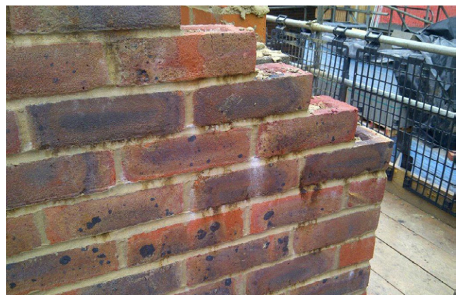
Staining on saturated brick work
