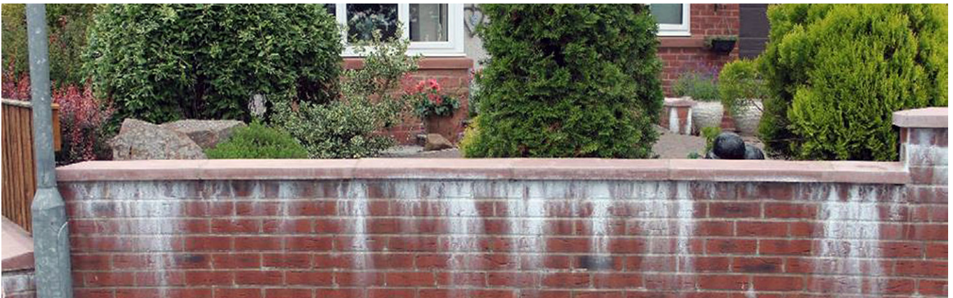
Lime staining caused by runoff from a concrete coping
