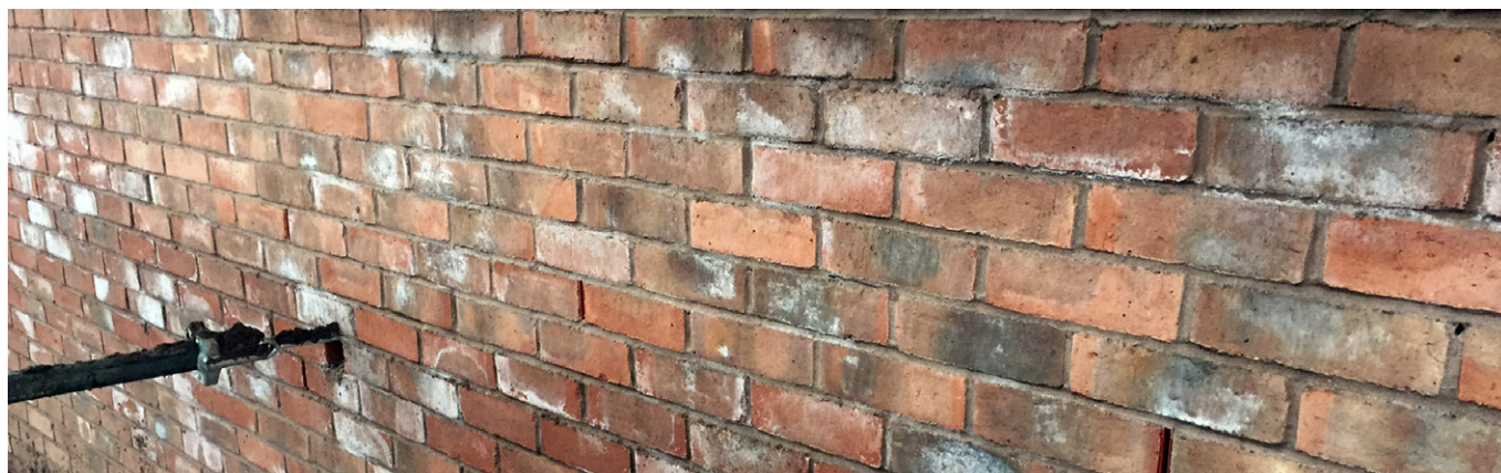
Efflorescence on brickwork under construction
