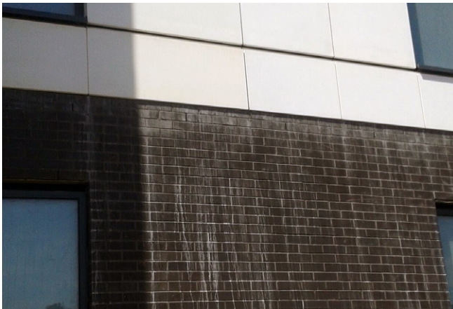
Staining from runoff over adjacent concrete components
