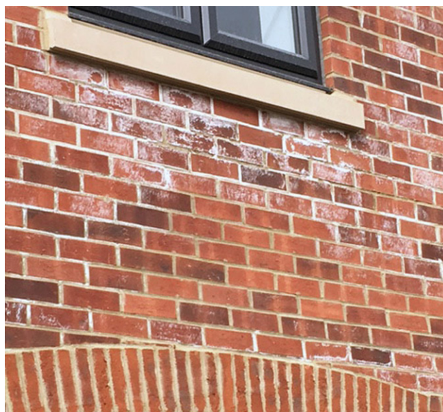
Efflorescence is the most common form of brick staining
