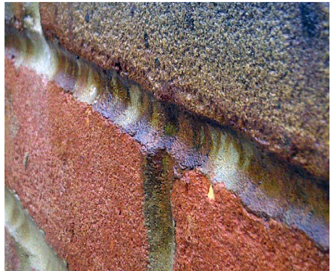
Iron staining visible on a mortar joint
