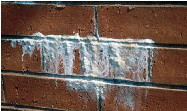
A severe case of lime staining
